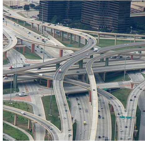
Figure 2: Complex grade separation
