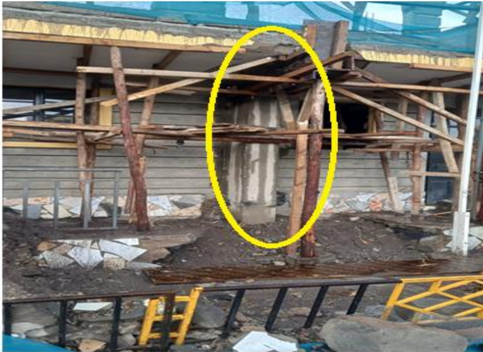
Figure 10: Independent columns carrying mid-slab beam loading as retrofitting remedial
