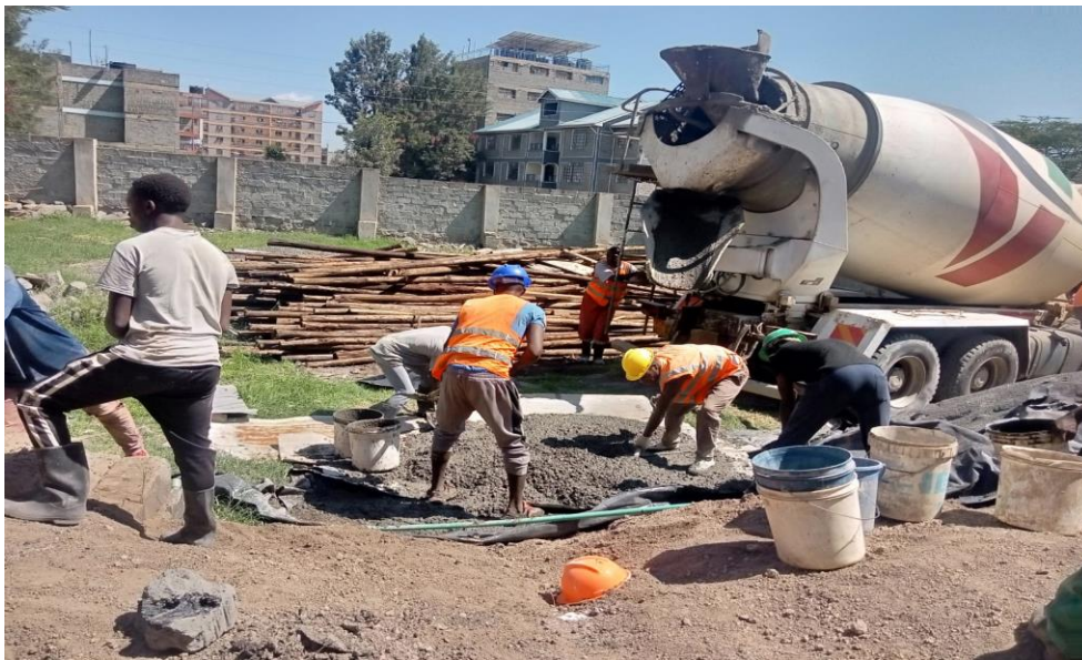
Figure 11: Purchase of ready-mix concrete from a reputable supplier to assure quality control
