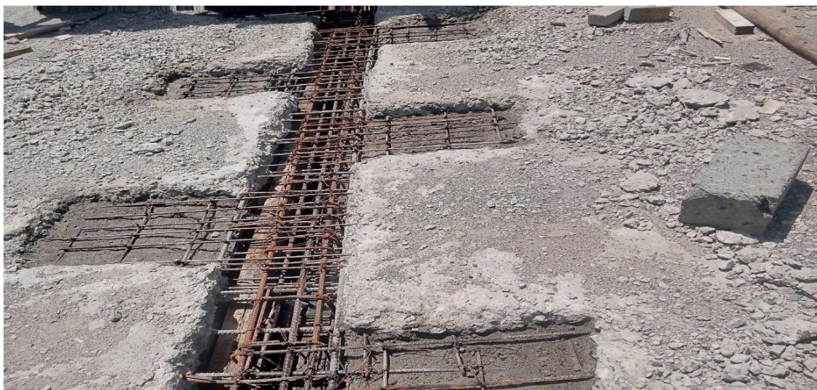
Figure 9: Supportive beam added mid-slab as part of the retrofitting remedials
