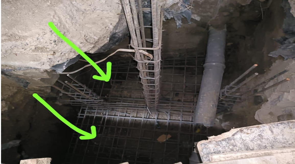
Figure 8: Structural members added as part of the retrofitting remedials
