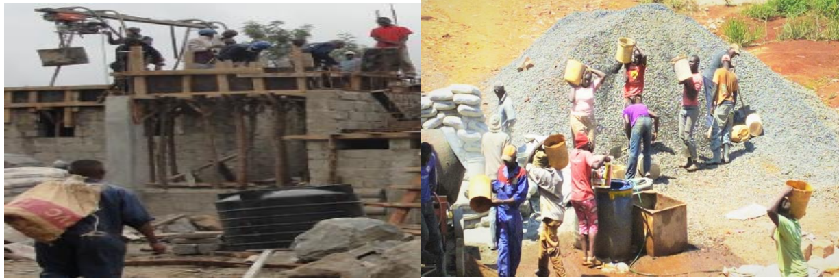
Fig 1.1: Concrete mixing gangs in a construction site (Ruaka, 2018)
