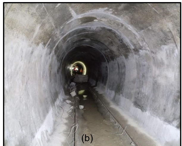
Figure 1: (a) shows the NCT crossing four rivers, (b) concrete lining of NCT tunnel
